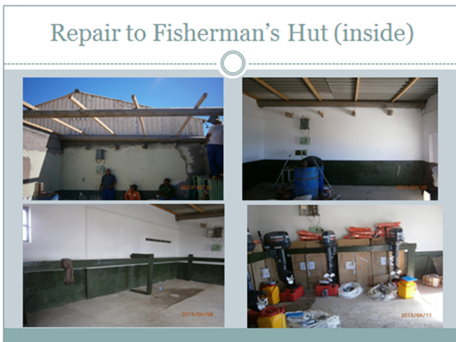
Fig 3: Repairs to Fisherman's hut in Hondeklipbay
